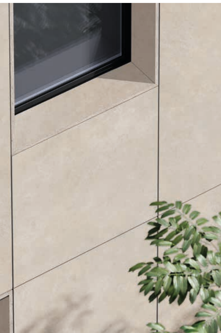
window sill ABKSTONE limestone greige nat 12 mm facade ABKSTONE limestone greige nat 6 mm
